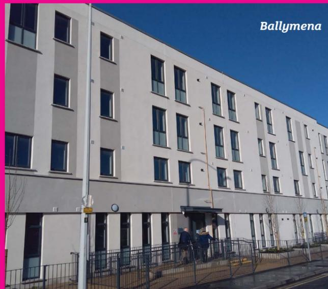
The building was previously used as a government office and was fully refurbished to deliver the apartment scheme. This involved the demolition of internal and external structures of the former building, stripping it back to the core steel frames and concrete slabs and constructing updated internal layouts, including dividing the building into two distinct blocks, as well as new external walls and façade.
